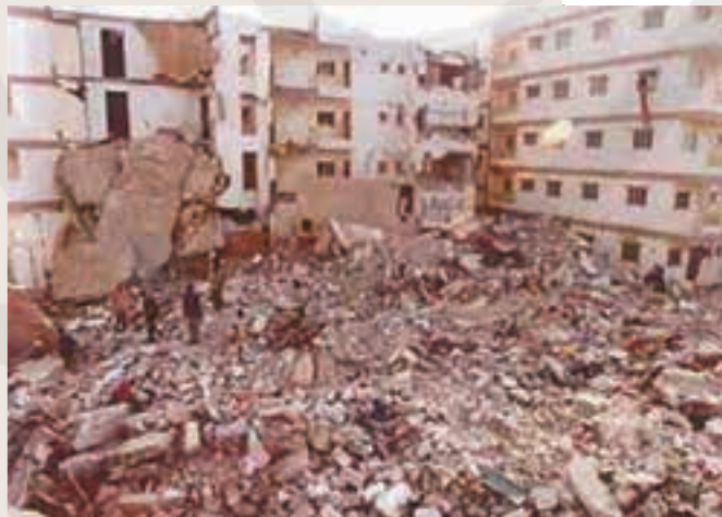
Fig. 2.5. The extensive damage caused by the major earthquake in Gujarat in 2001
